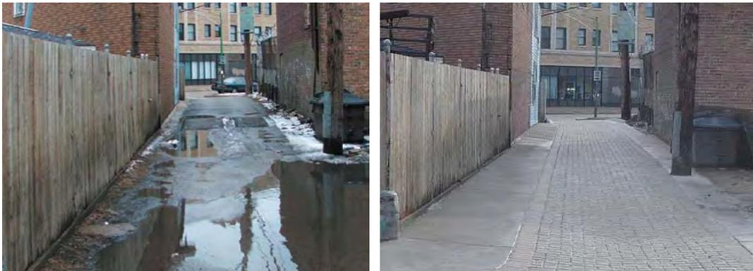
**Figure 17. Alley with impervious pavement and poor drainage (left); alley with pervious pavement resulting in no standing water (right).**
