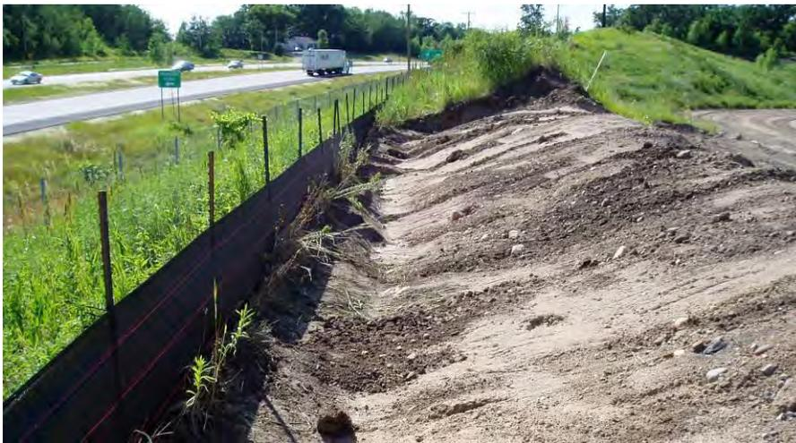
**Figure 27. Installed silt fence will minimize sediment from leaving a site and entering surface waters.**
