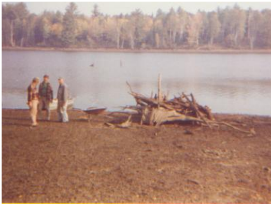
Building a fish crib during the draw down on Lake Alice -- September 1983.
