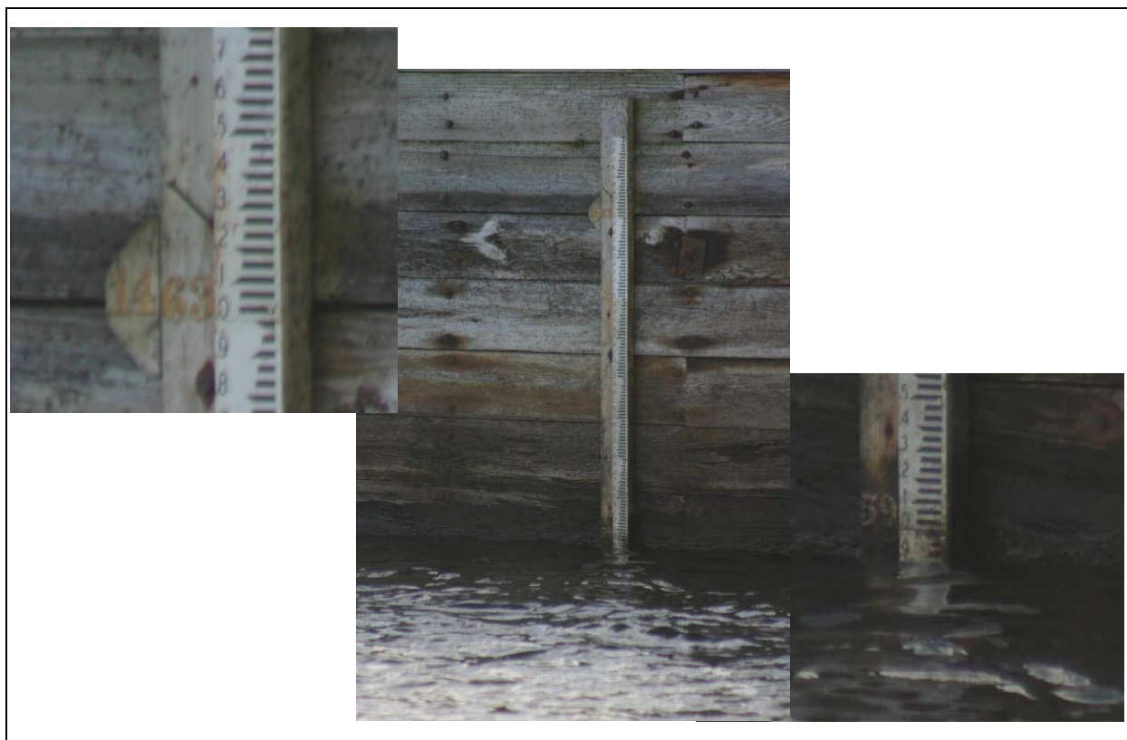
Photo 2. Nokomis (Bradley) Dam staff gage. Center picture shows full gage as it is mounted on dam. Left picture shows close up of nail marking maximum level of 1463.25 feet above MSL. Right picture shows close up of water level reading of approximately 1458.80 feet above MSL on the day the picture was taken (November 12, 2007).
