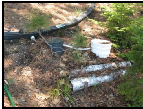
F) 5-gallon pail added to increase capacity
