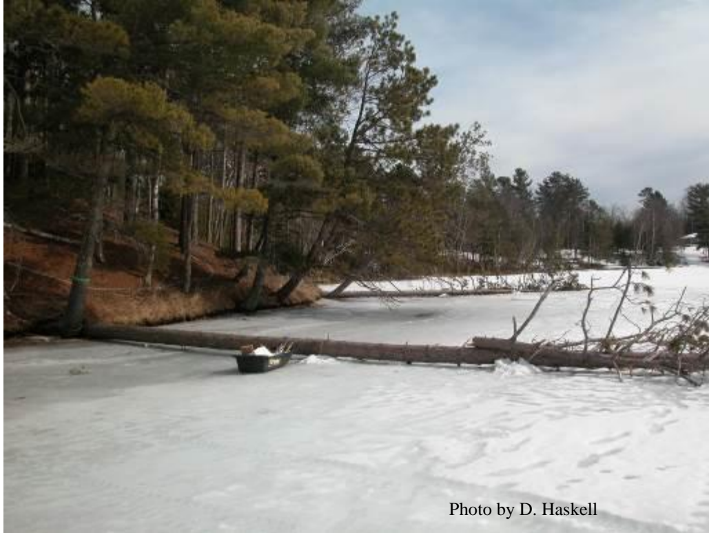
Figure 27 Tree drops installed at Lou Mirek’s Property on LSG Lake during the winter of 2011. Trees were later secured to lake bed using steel cables and earth anchors.
