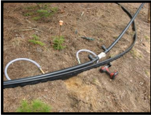
A) 2" ABS pipe connected end-to-end
