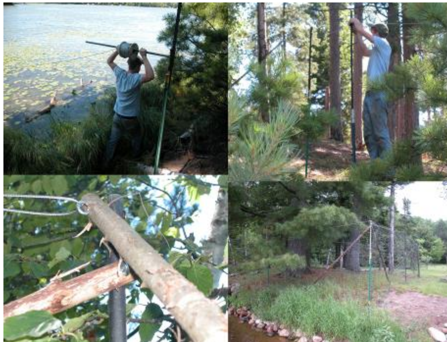
Figure 28 Construction of deer abatement fence on LSG Lake in 2011-2012.
