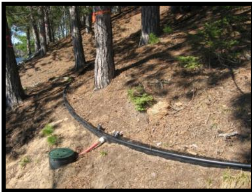
E) Completed installation (plot L)
