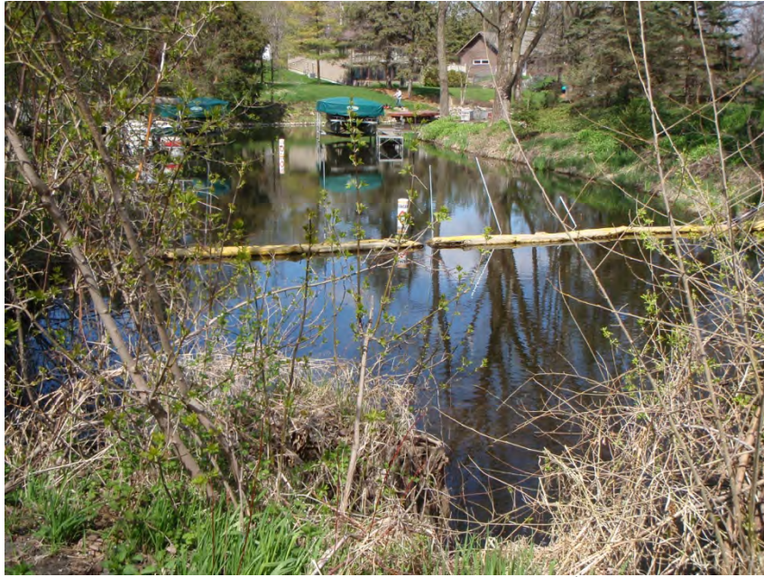
Figure 6. Turbidity barrier in Miljala Channel
