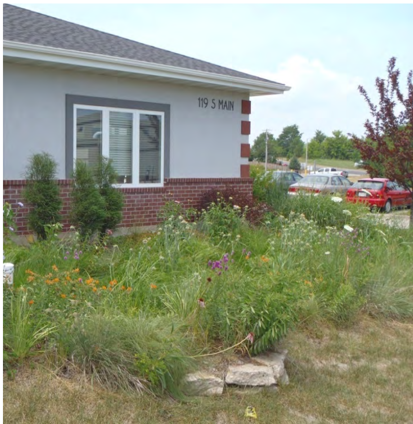
Figure 8. Rain garden capturing roof runoff.
