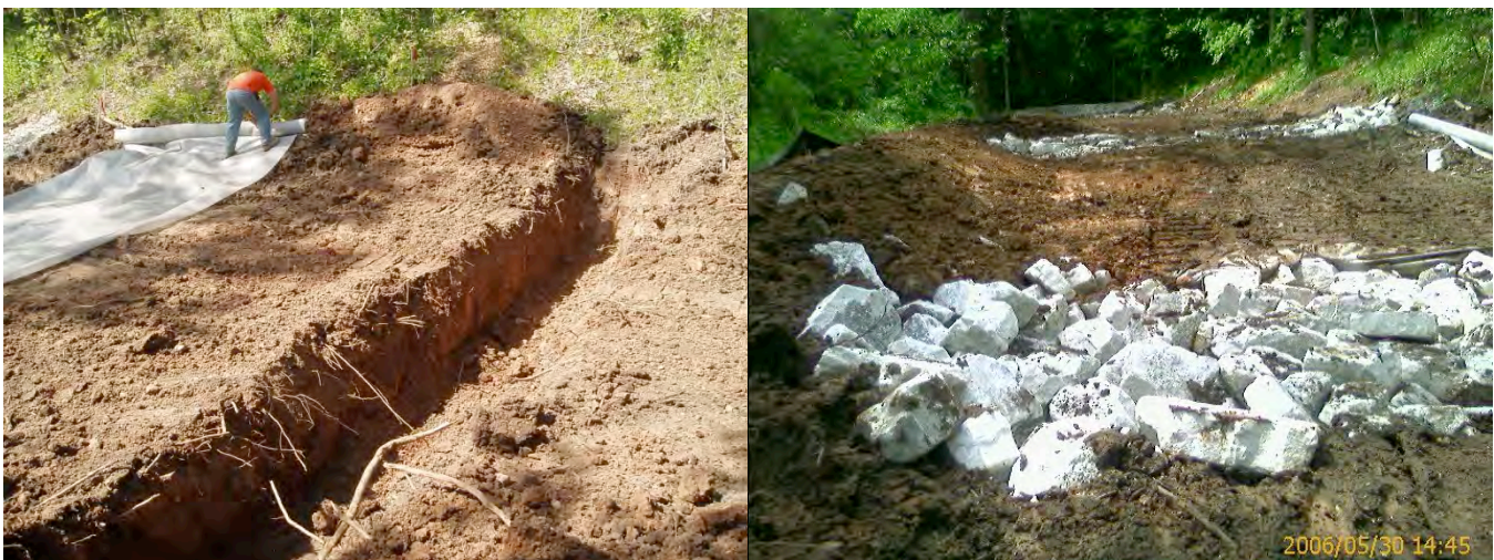
Figure 12. Example of rip rap grade control buried in channel bed.
