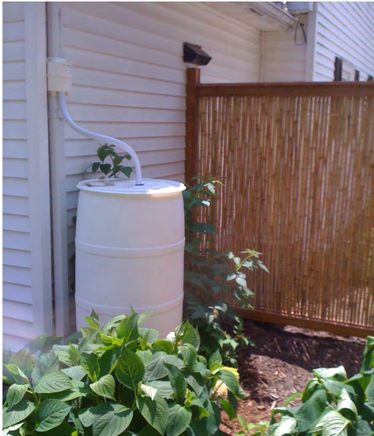
Figure 9. Rain barrel capturing roof runoff (from Sustain Dane)
