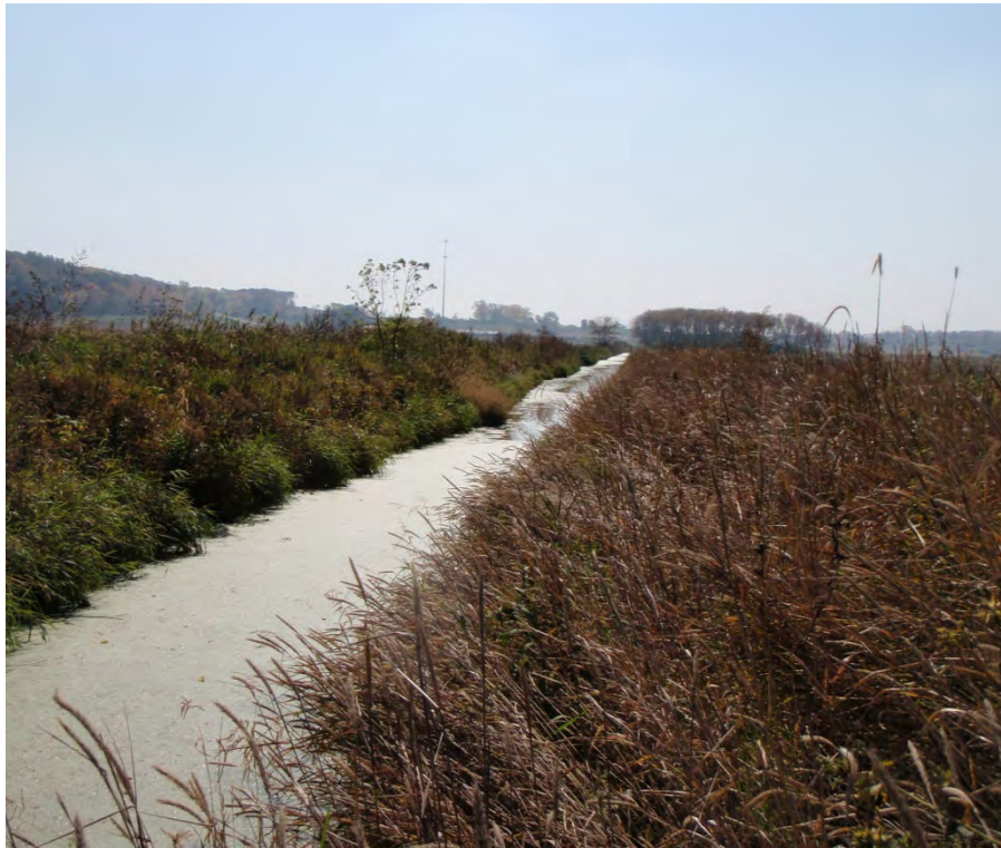
Figure 11. Ditch with right bank recently re-sloped and planted with grass. Left bank not stabilized.
