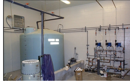
Alum is stored in the pictured tank (above). The phosphorus remains in this pond (below).
