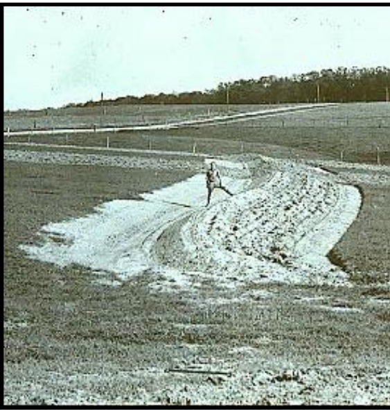
Figure 6. Installation of a field terrace on a coulee region farm circa 1934.
