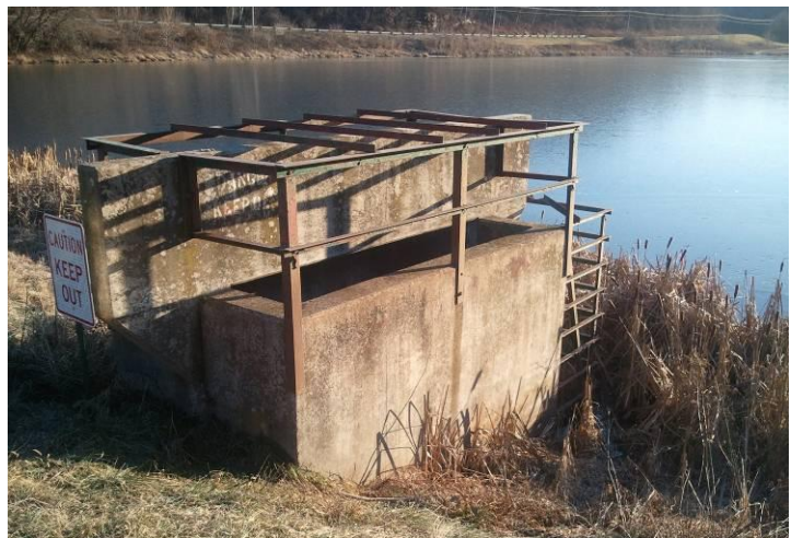
Figure 1.4. Existing dam control structure
