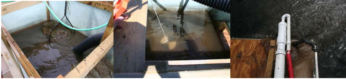
Figure 12. Water with a relatively high sediment load flowing through and off the HCS.
