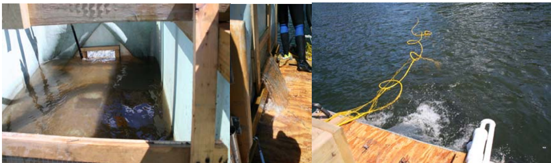
Figure 11. Relatively clean water flowing through (left and middle) and off (right) the HCS.
