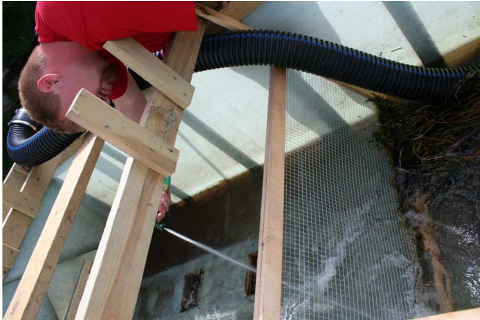
Figure 10. HCS crew hosing of the screen of the primary containment area.
