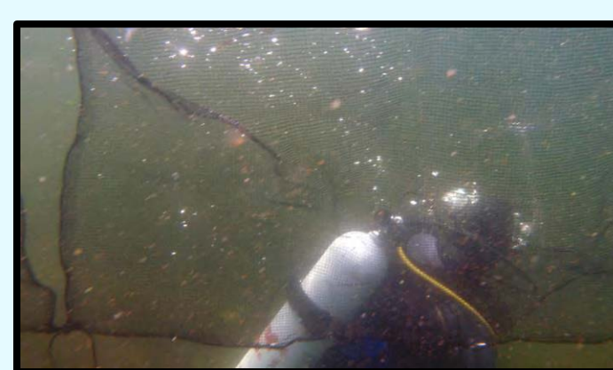
SLA diver installing the Fragment Barrier
