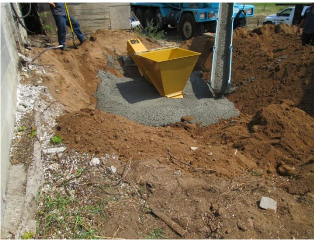
Manure pump installation.
