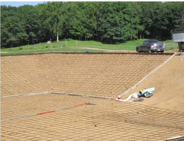
Installing concrete re-bar reinforcement
