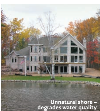
Unnatural shore – degrades water quality
