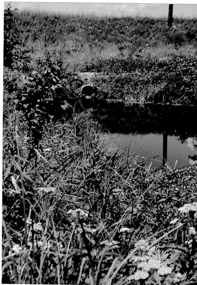
Tomahawk Earth Dam Drain Outfall.
