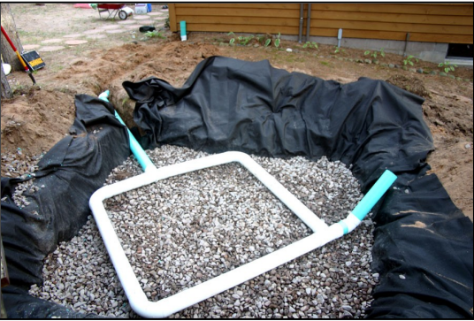
Infiltration Pit Under Construction
