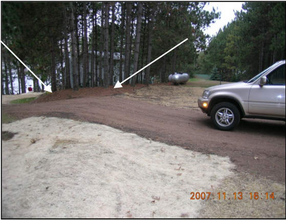
Berm Keeps Water from Eroding the Slope to the Lake
