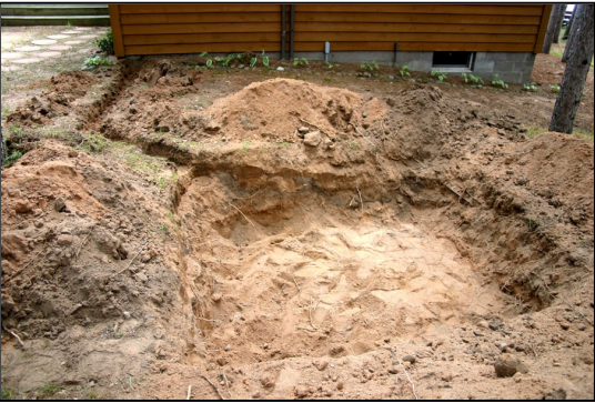
Infiltration Pit Dug to Capture Roof Runoff Water
