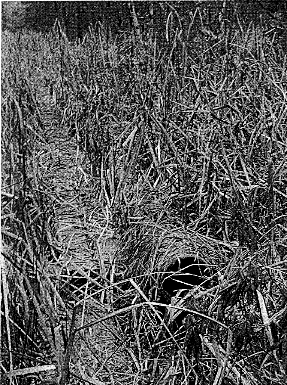
Figure 8. Drummond WWTF dispersal pipe in bog wetland – no visible discharge.
