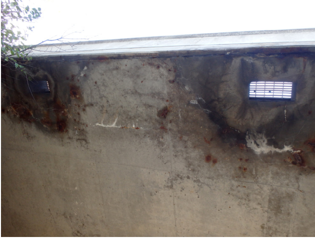
Figure 10 DRAINAGE FROM IH 94 OVERPASS
