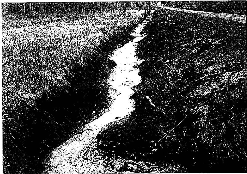
RECENTLY EXCAVATED LATERAL DITCH CONNECTING TO TRIB.
