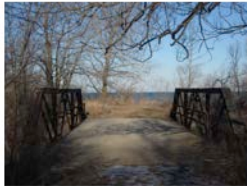
Fischer Creek – Company in Indiana
