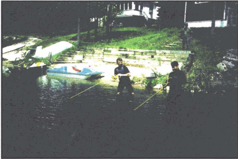
Figure 13 PULLING IN ROLL OUT BENTHIC BARRIER
