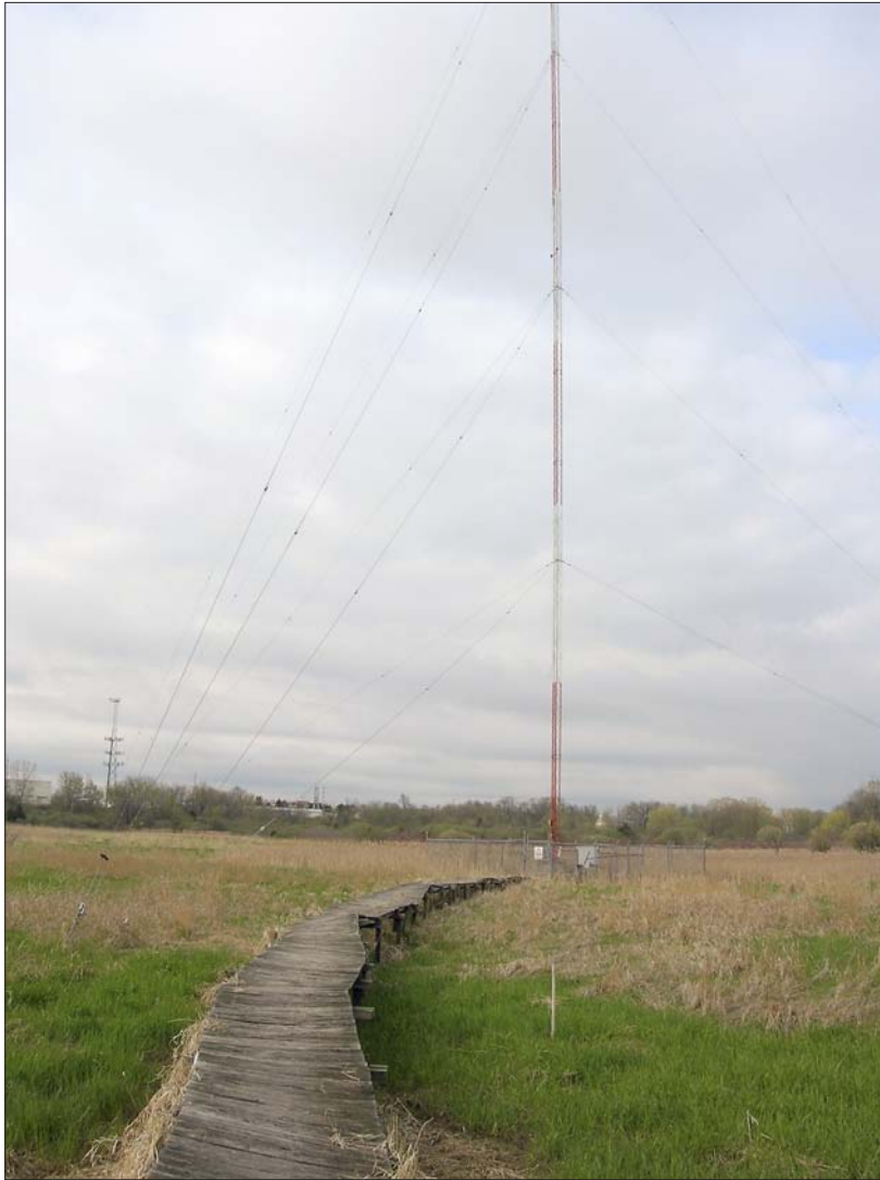
Figure 2.9: The WHA-AM radio transmission tower in the background of Southeast Marsh.
