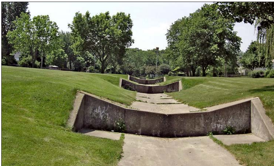
Figure 7.4 View of the Arbor Hills Greenway and the existing drop structures.
