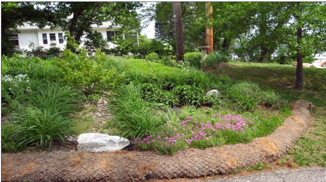
Figure 15.4 An example of a residential rain garden. Source: Wisconsin Department of Natural Resource. http://dnr.wi.gov/runoff/rg/RainGarden_genl_newsletter.pdf
