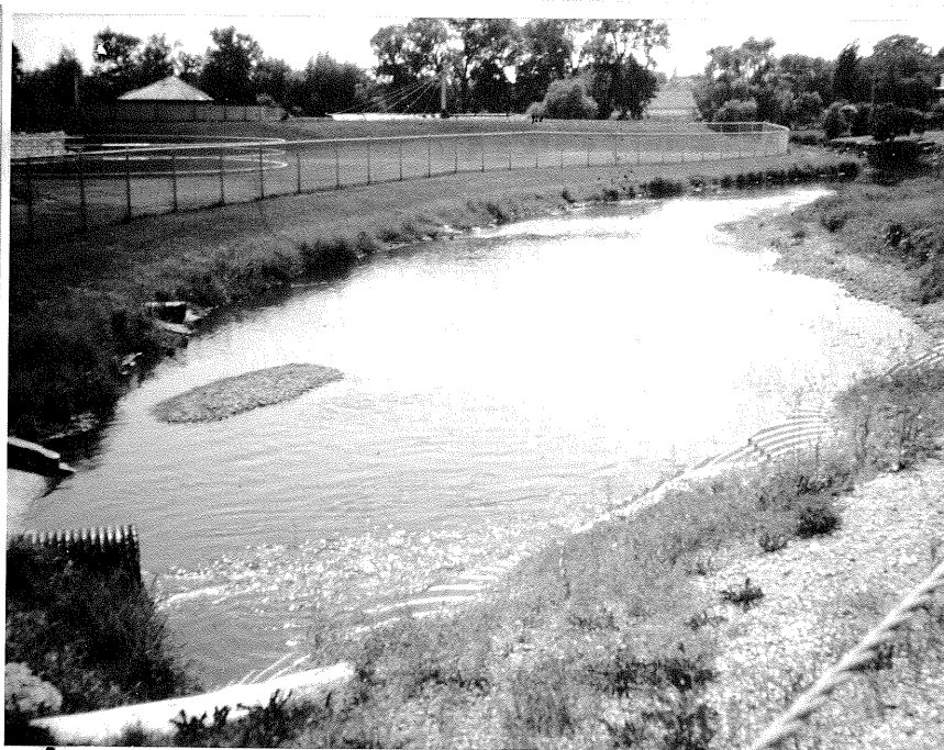
Beaver Dam - STP and Outfall
