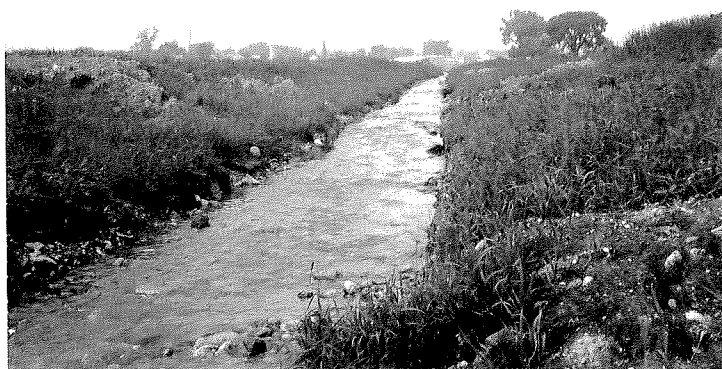
Constructed effluent channel carrying Elkhorn's treated wastewater
