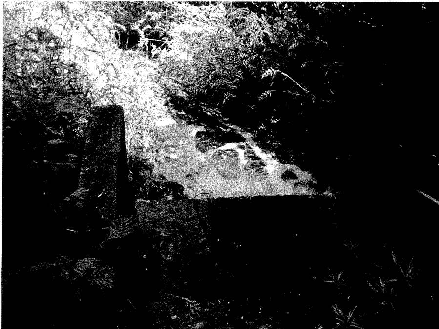
Slinger WWTP outfall looking North
