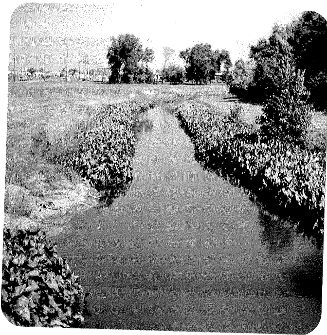
Neenah Slough looking downstream from Cecil Street bridge in Neenah.
