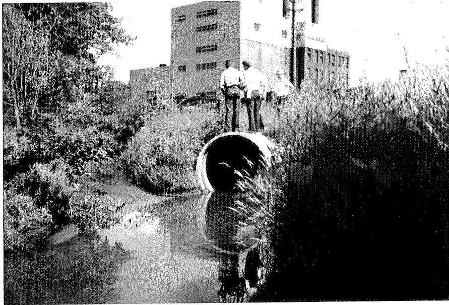
Storm sewer outfall, headwaters of Mill Creek
