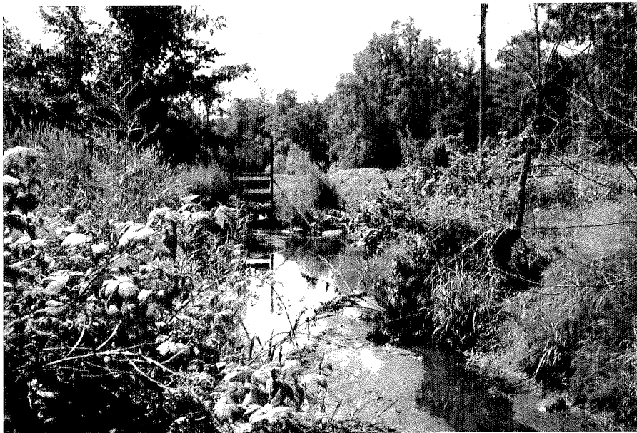
Downstream from storm sewer outfall
