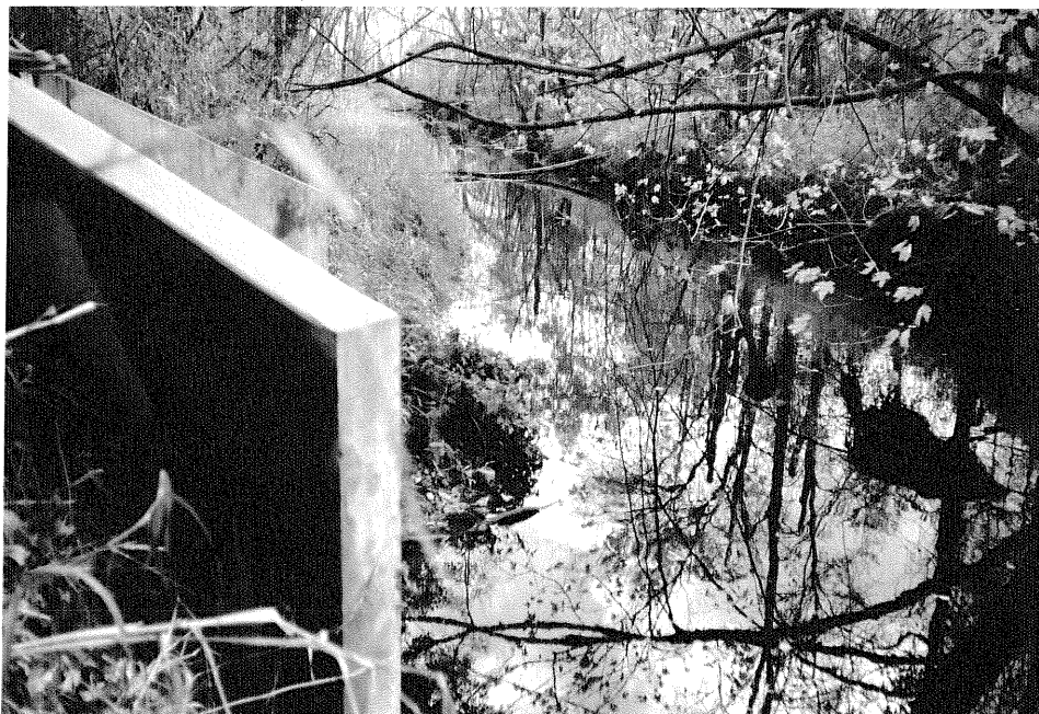
Hewitt Outfall Structure to Mill Creek
