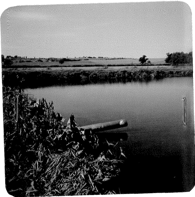
Roberts WWSP - second cell with discharge pipe, looking WNW
