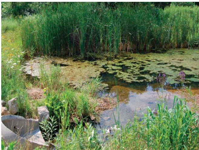
Photo showing stormwater drains outside of University of Platteville.
