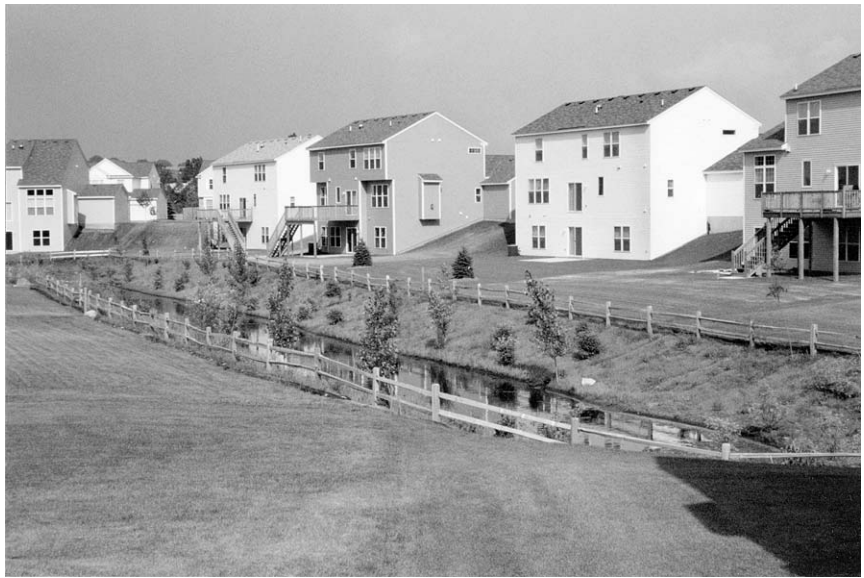
Figure 3.2. A bioretention pond with sand bottom in Earley Lake Estates, Burnsville, Minnesota (courtesy of Tara Roffler, University of Wisconsin–Madison, Water Resources Management).
