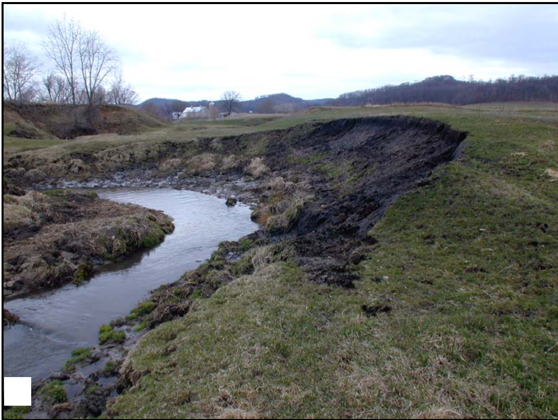
Figure A-7. Stream bank erosion located in middle section of stream.
