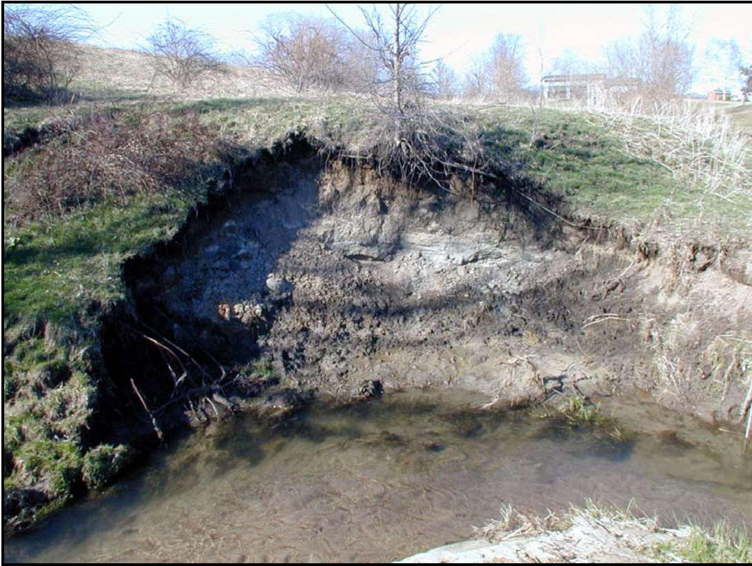
Figure A-10. Stream bank erosion located in lower third of stream.
