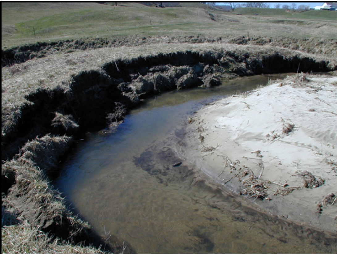
Figure A-13. Stream bank erosion located in lower third of stream.
