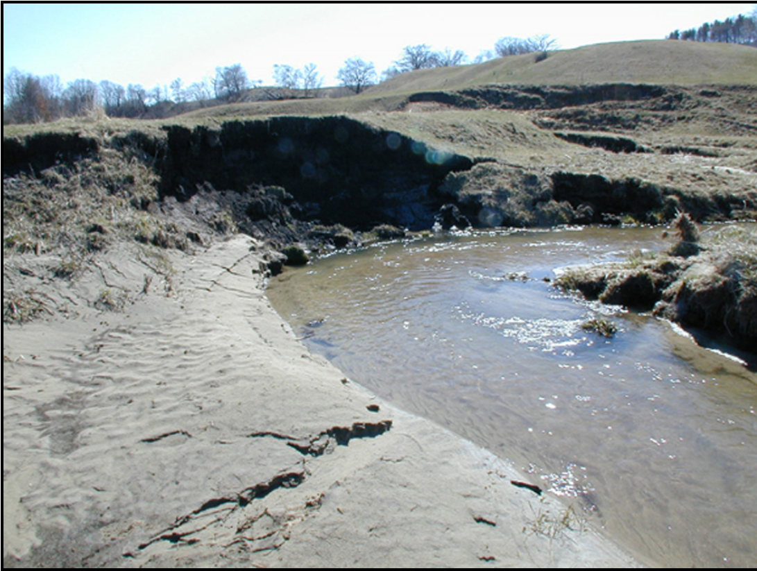
Figure A-12. Stream bank erosion located in lower third of stream.
