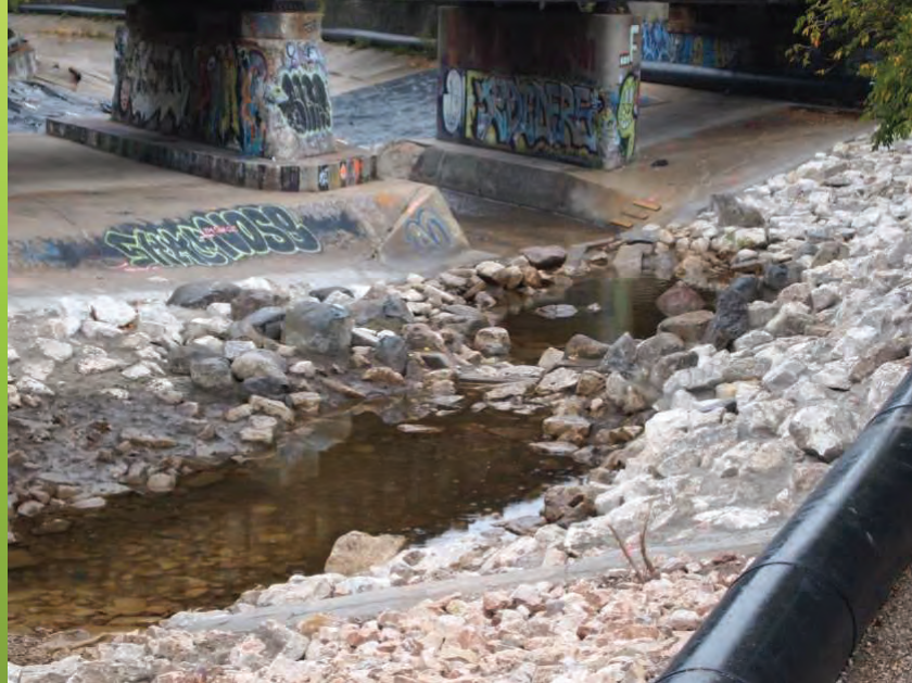
Upstream RR Bridge
