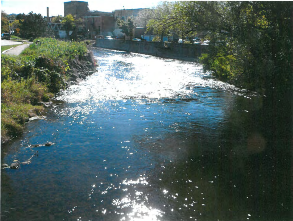
Photo 7. Erosion visible (top left) along Milwaukee River.
