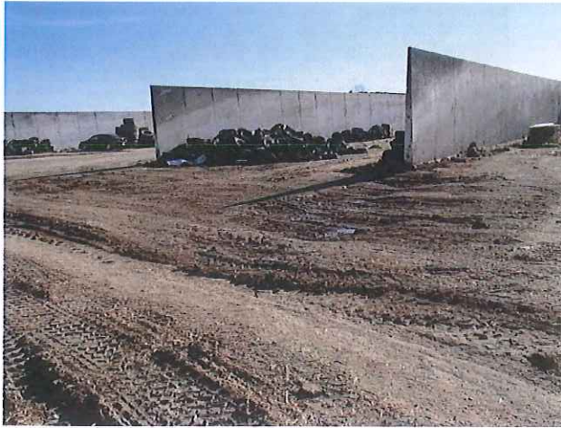
Concrete pad to be removed
