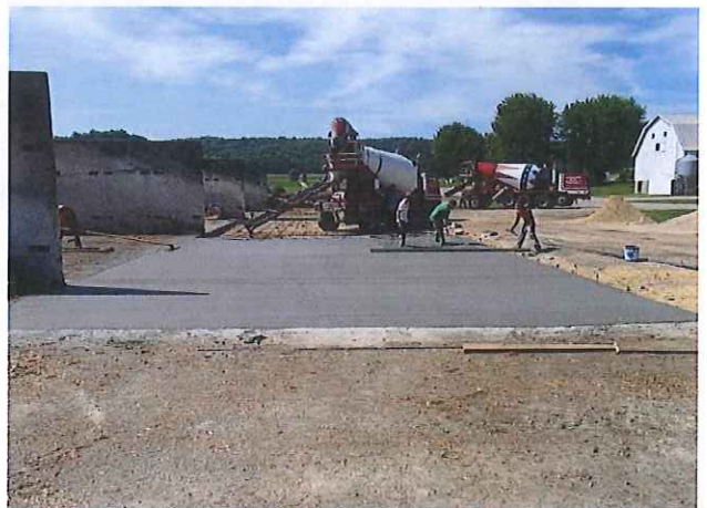
Placing concrete
