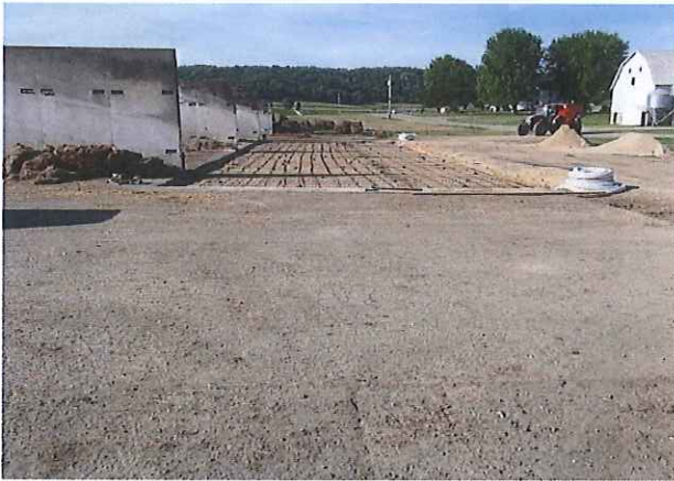
Concrete pad removed with tile being installed
