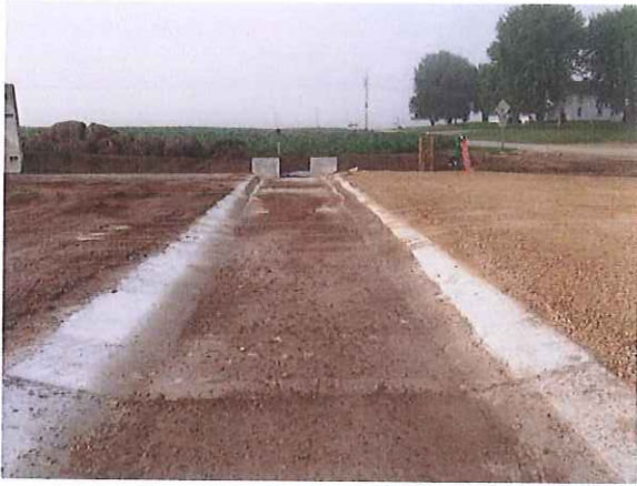
Channel looking south with screen
