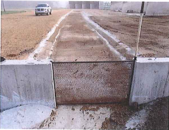
Channel looking north with screen
