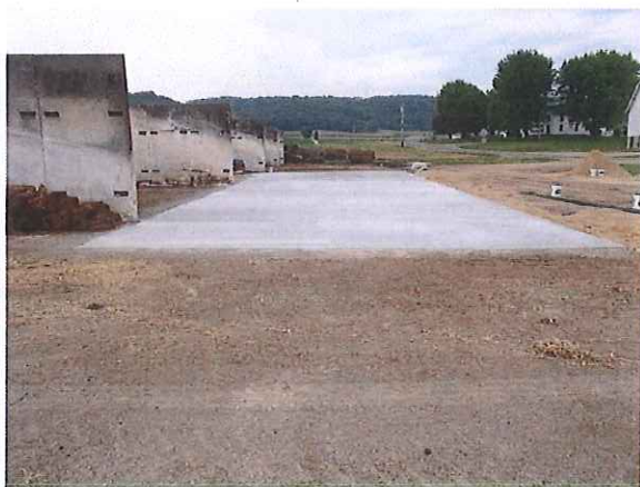
Concrete pad installed
