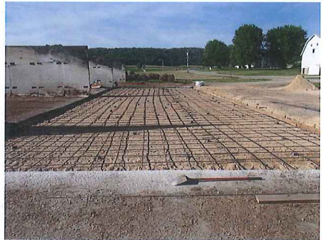
Concrete pad removed, rebar installed
