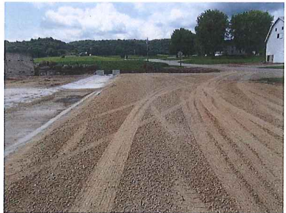
Gravel installed west of channel looking south
