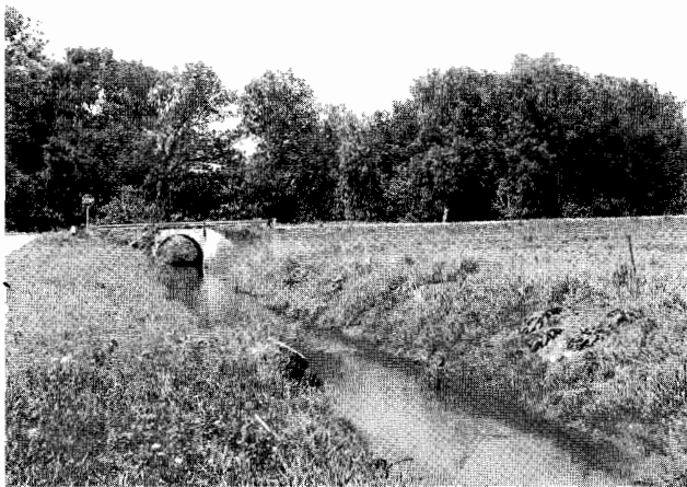
In the past stormwater systems were designed to remove water as quickly as possible
