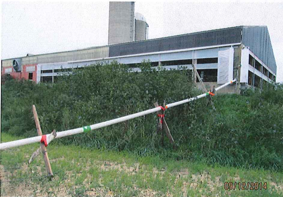
Photo 2: South end of temporary manure transfer system from the barn to manure storage. Preisler needs to repair the manure transfer systems and stop using the temporary transfer pipe.
