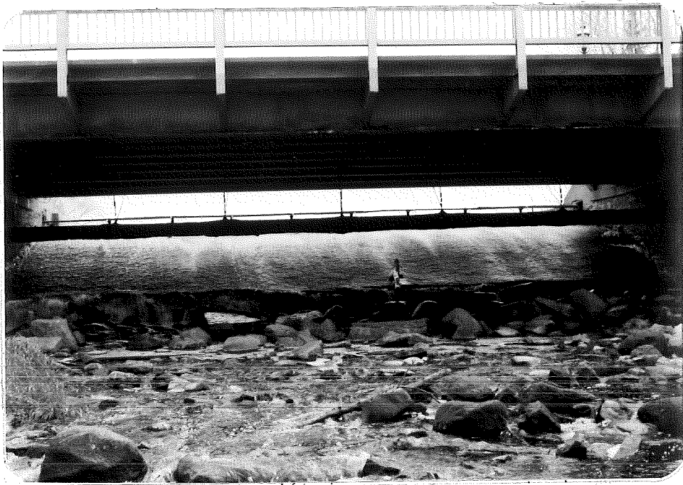
Black Otter Creek looking upstream toward the dam (4-30-81).
