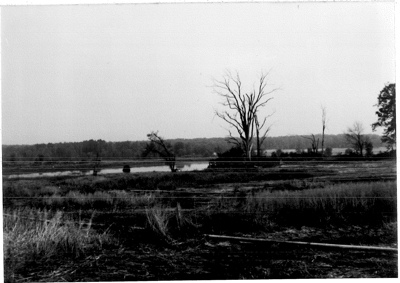
Larsen Company spray irrigation field looking SE past the lagoons. The wastewater is sprayed onto this field and then allowed to drain into the lagoon in the center of the photograph. Note the large amount of dead vegetation resulting from wastewater overloading of the field. (September 7, 1982).
