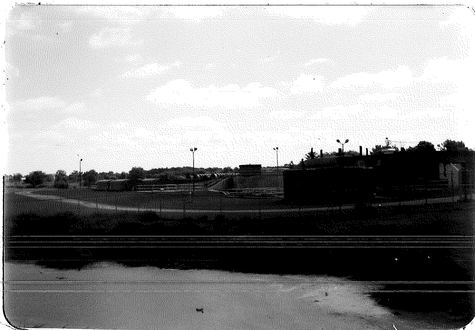
Village of Black Creek POTW looking SE from Hwy 55. The effluent discharged is in the center of the photograph. (September 3, 1981).
