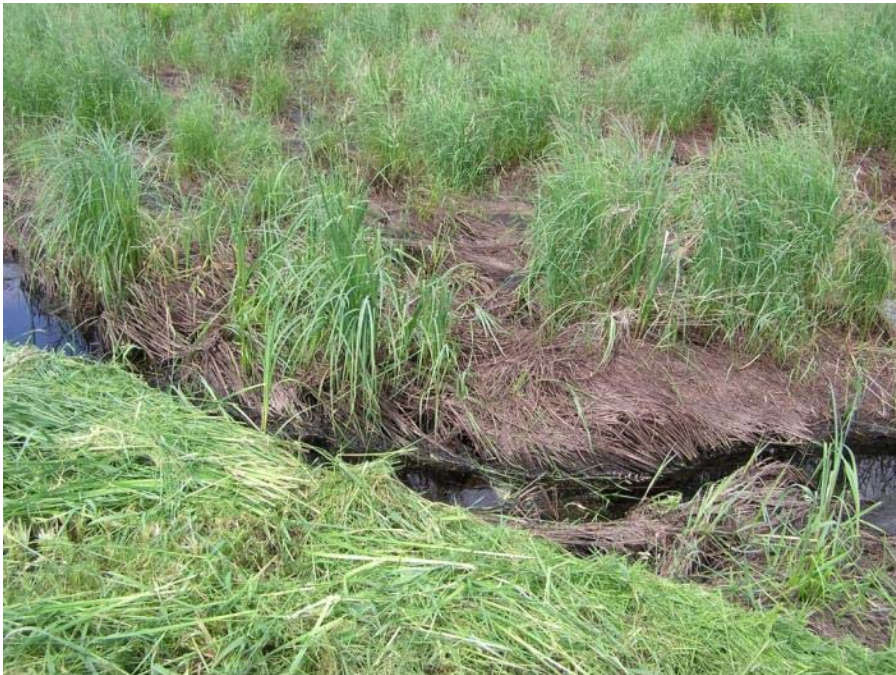
Figure 24. West ditch along Lundquist Road
