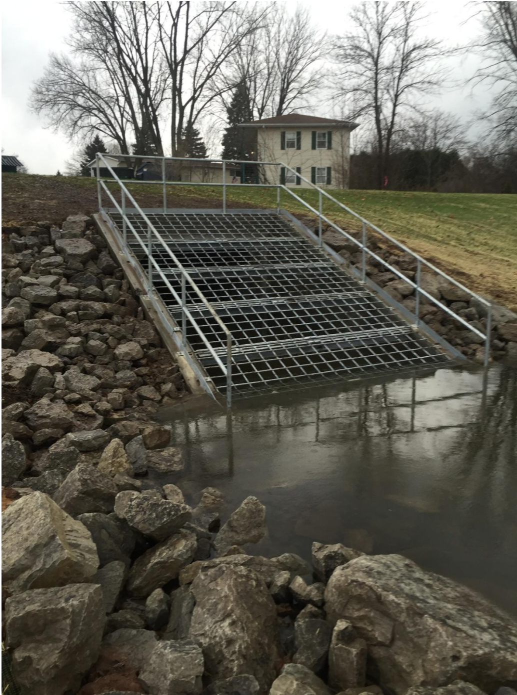
Picture 2 is the completed inflow structure at south end of the basin.
