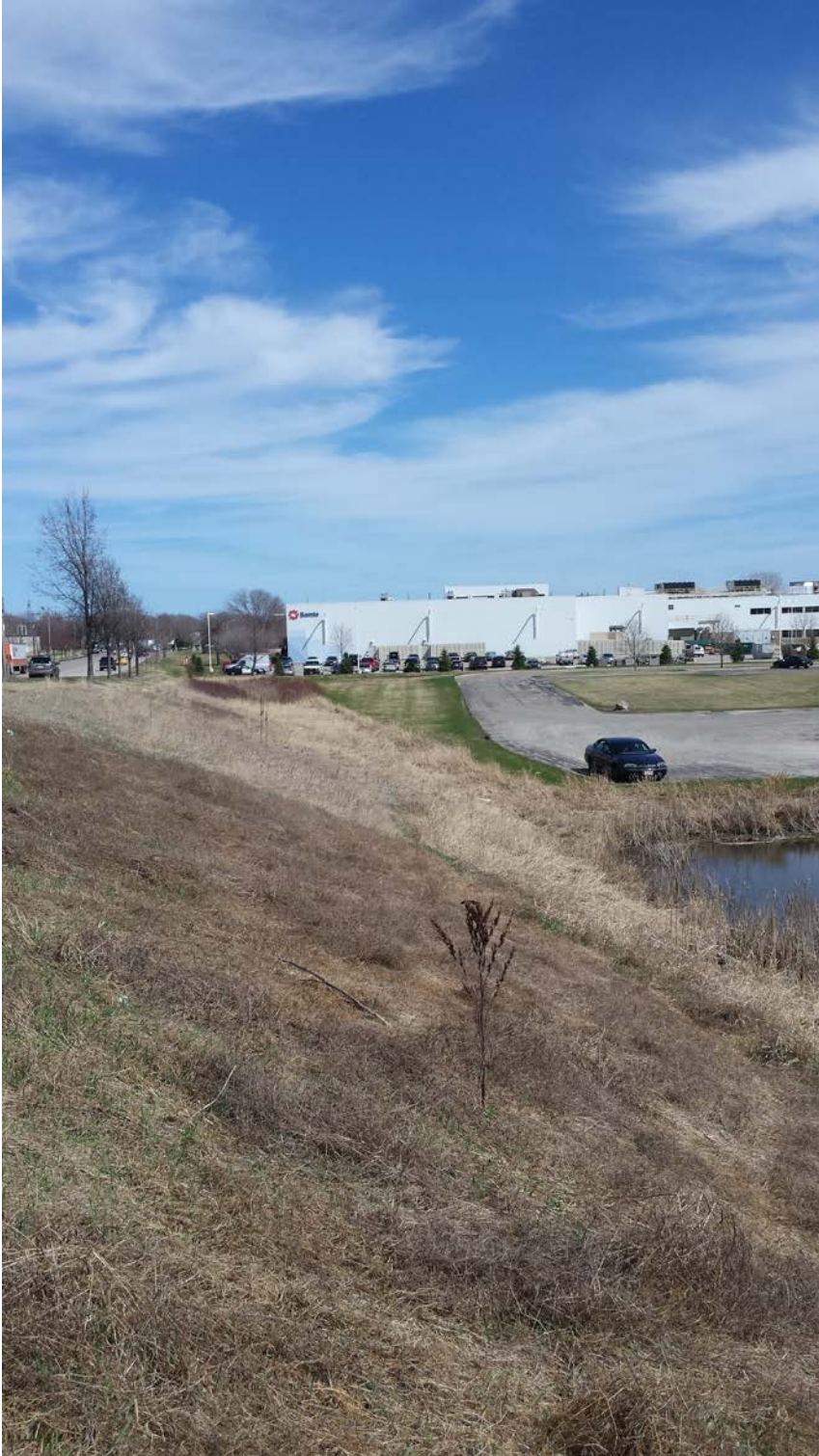
Area of Storm Sewer Installation at Pond Looking East
