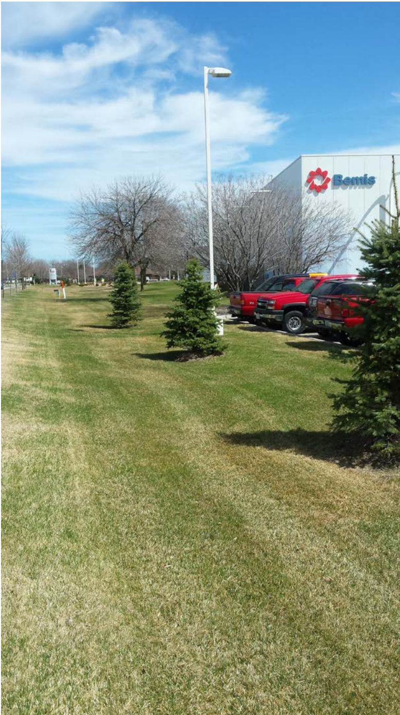
Area of Storm Sewer Installation Midway Looking East
