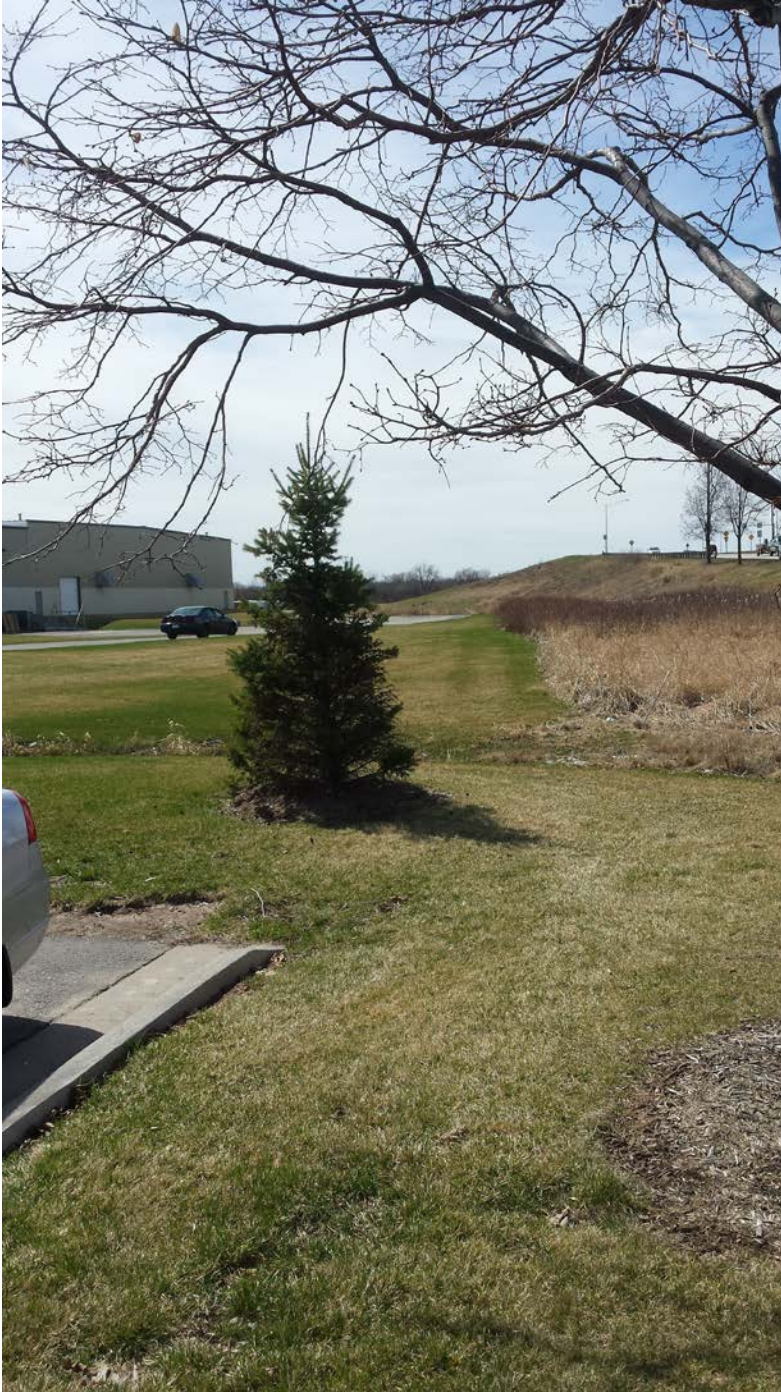
Area of Storm Sewer Installation Midway Looking West
