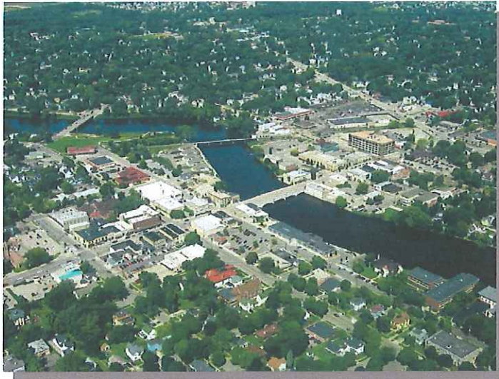
The Rock River weaves through downtown Fort Atkinson
