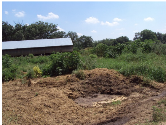
Unlined manure storage.
