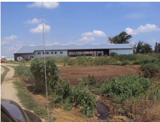
Unlined manure storage.
