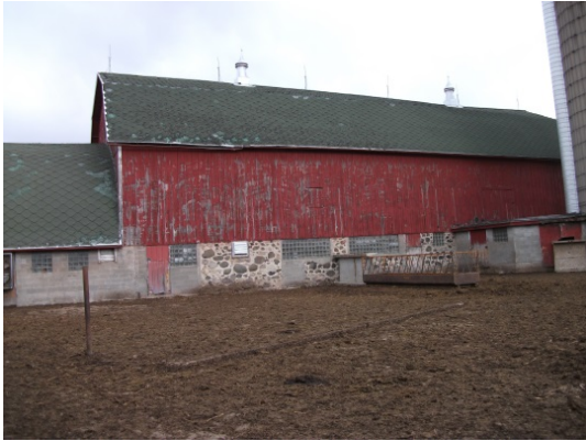
Barn before gutter installation
