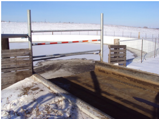
Manure transfer system
