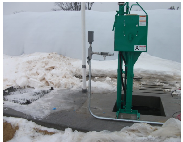
Feed leachate waste transfer tank, pump
