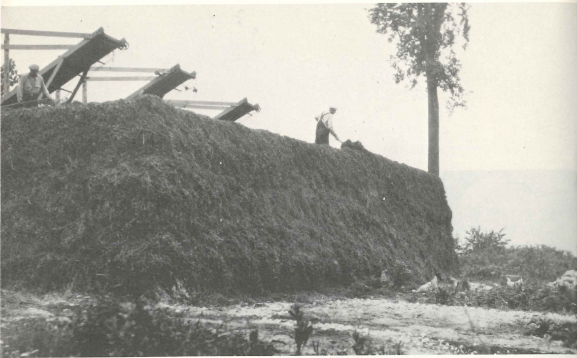
Leaching from pea vine stacks used to be a common cause of both surface and groundwater pollution.
