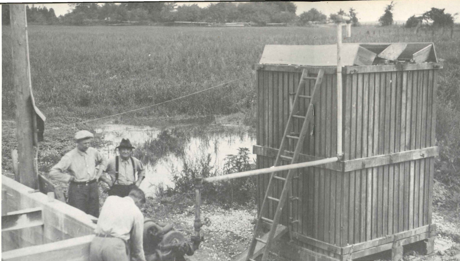
This experimental trickling filter was one of many research projects which were helpful in improving waste treatment technology.
