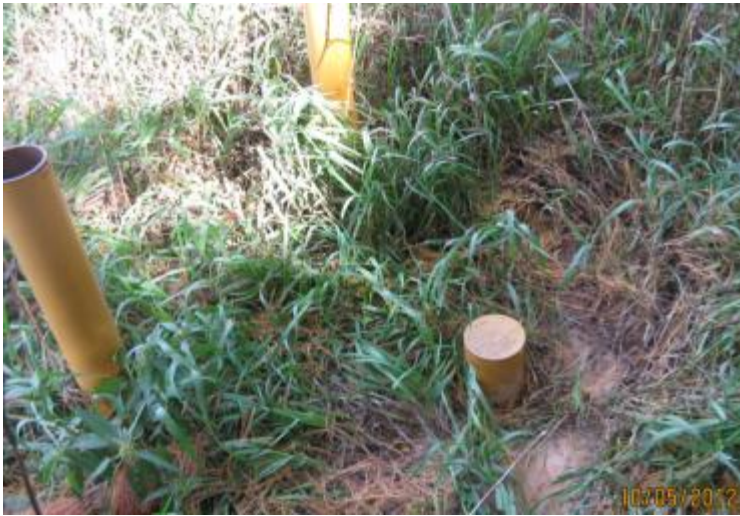
Photo above well GL1-1, either well has settled or runoff from lot shown on right has filled in ground around well. Photo right is looking northeast at lot 2.
