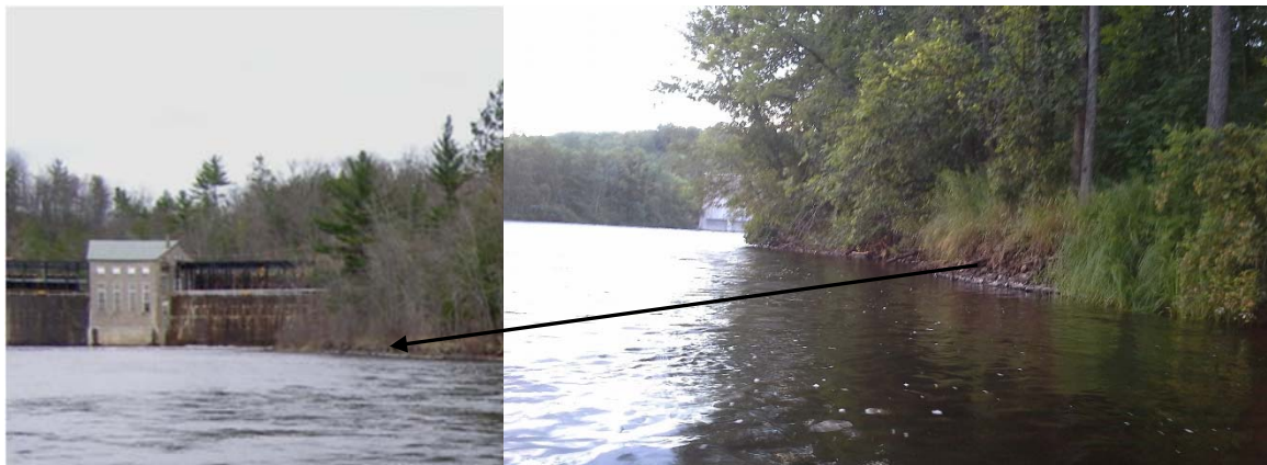
Photo taken from the site and looking toward the dam looking upstream toward the dam.
