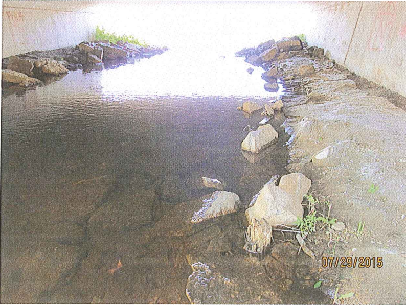
Photo 3. Ogden Street Bridge S Channel Menominee River - Facing East
