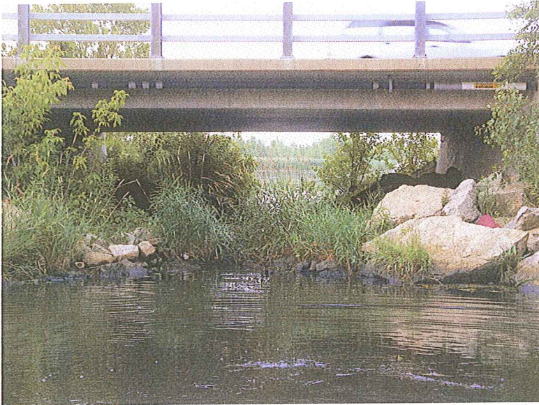
Photo 1. Ogden Street Bridge S Channel Menominee River - Facing East
