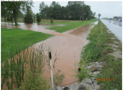
Looking southwest at field runoff entering the culvert on the south side of State Road 54. A large volume of sediment-laden water was entering the Dax farm due to very heavy rain at the time of the site inspection.
