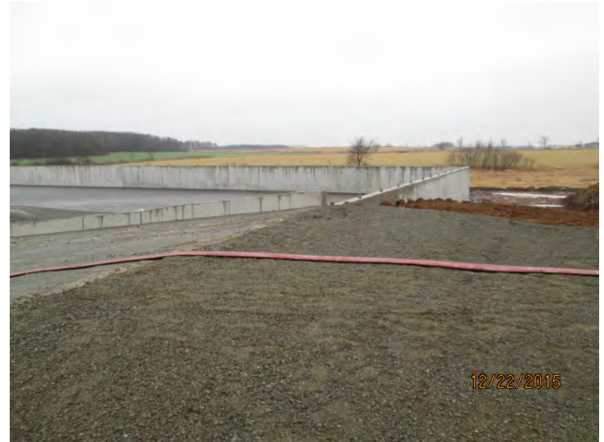
Looking south to north at new waste storage facility
