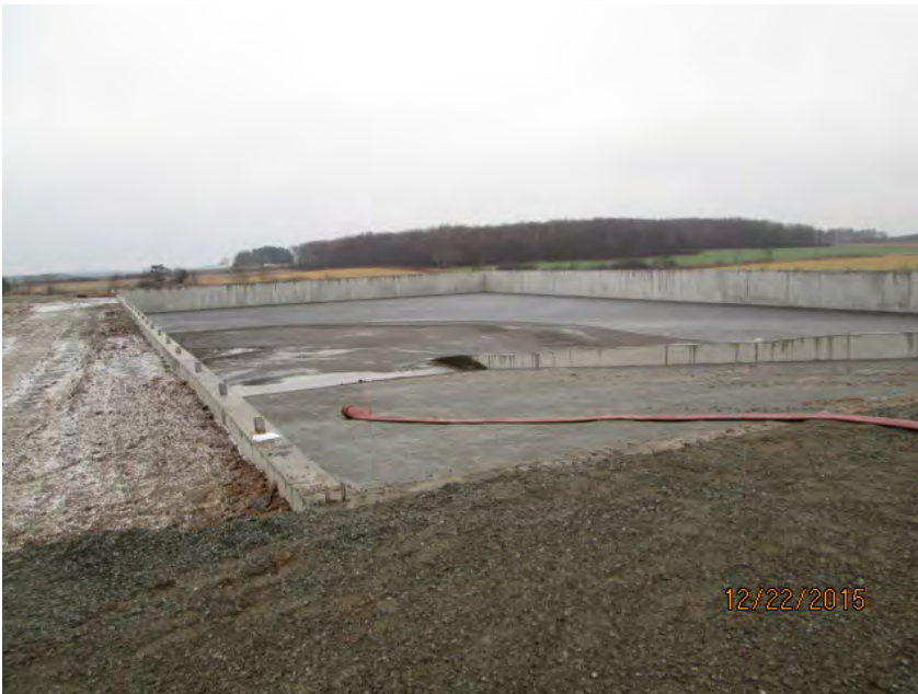
Looking east to west at new waste storage facility
